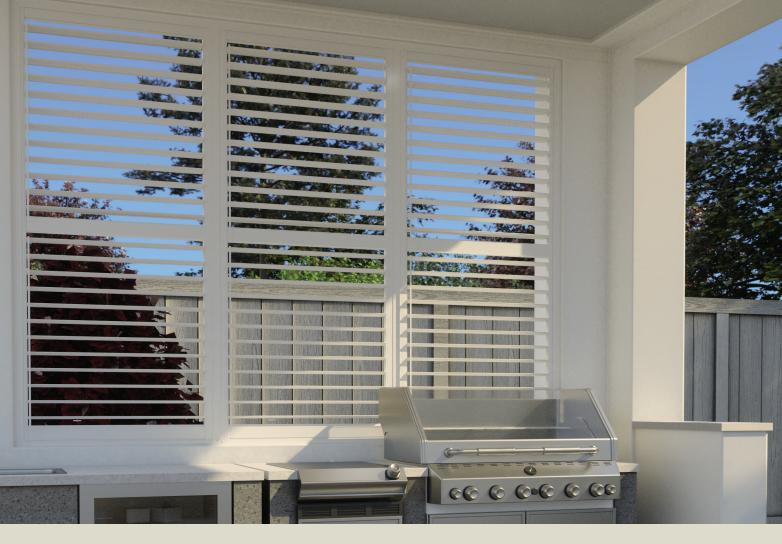
Aluminium shutter panels are custom made to size and arrive fully assembled. Tilting louvres open gives visibility and also lets a breeze pass through providing heat reduction. Closing louvres ensures privacy and reduces impact from the elements such as wind, sun and rain.
