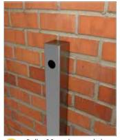
Drill a 25mm diameter hole through front wall of post
