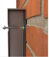
Drill rear wall of post with required diameter for fixing and then fix post to wall. Insert appropriate fixing into the wall for affixing post
